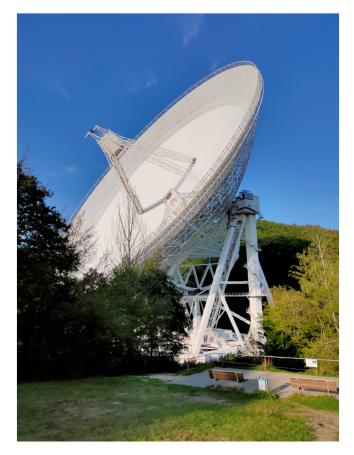
Figure 3.1: The Effelsberg 100 m telescope, located in Effelsberg, Germany, is one of the largest steerable single dish radio telescopes on Earth. With its 100 m dish it achieves high sensitivities and high angular resolutions.
