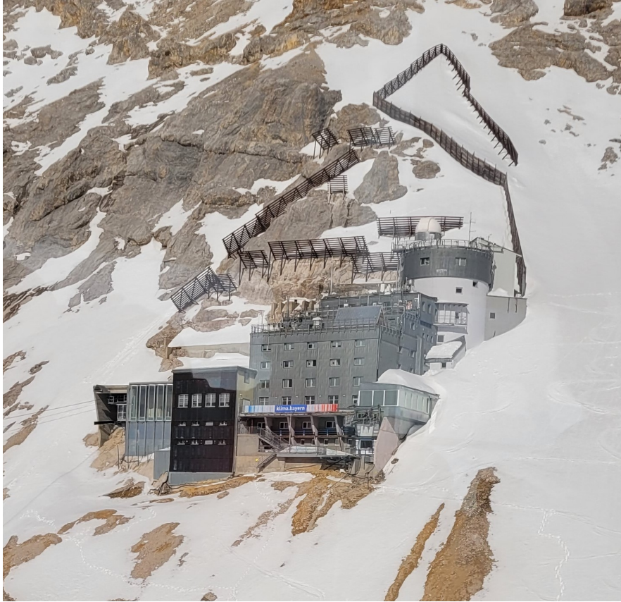
Fig. 4.1: The UFS located at the mountainside of the German-Austrian alps. It consists of several measurement platforms consisting of concrete. Several institutes collaborate to this research station.
