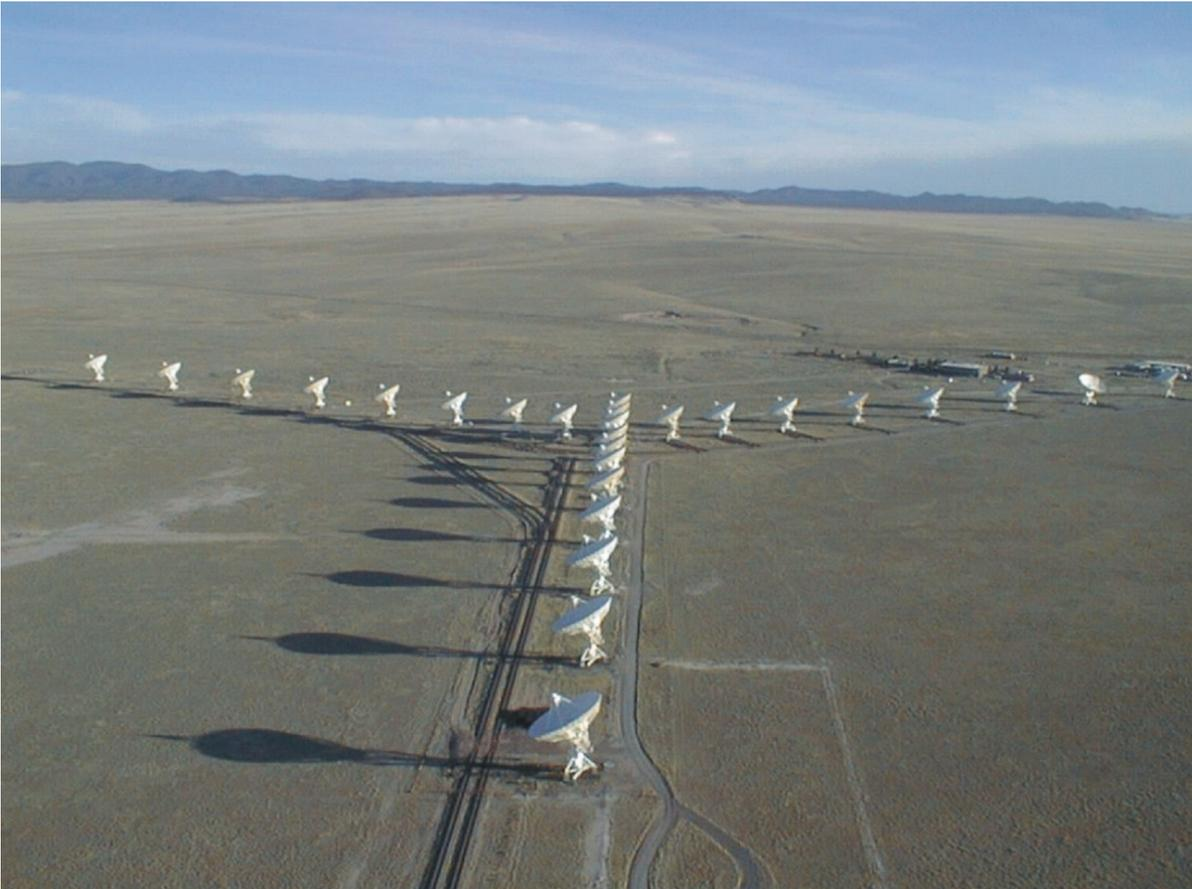
**Figure 1.9.:** Image of the whole VLA at D-configuration with maximal baselines of 1.03km. *Credits: Image courtesy of NRAO/AUI*
