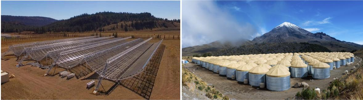
**Figure 3.1.:** *Left:* The four cylindrical parabolic reflectors that make up the CHIME radio telescope. Each reflector is 20 m wide and 100 m long. *Right:* The water tanks of HAWC, which are used to detect VHE  $\gamma$ -ray emission.
